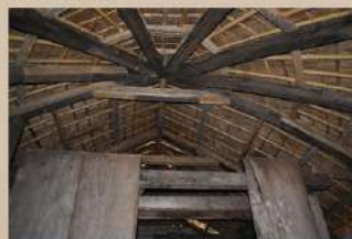
Fig. Roofing system in Khasi house
