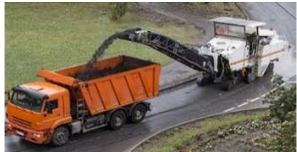
Figure-3: Milling of RAP material (Source: dykespaving.com)
