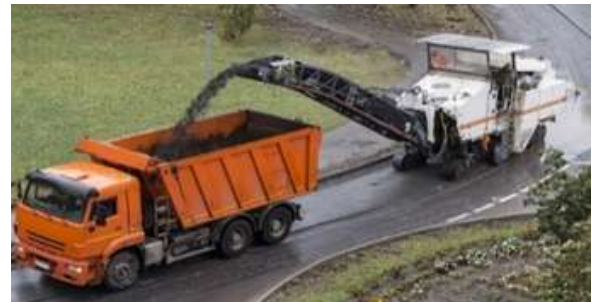
Figure-3: Milling of RAP material (Source: dykespaving.com)
