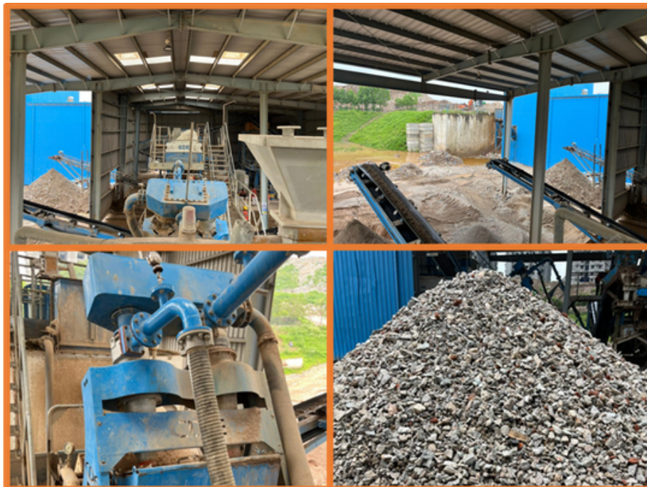
Fig. 2: Ramky C&D waste recycling plant in Hyderabad and recycled aggregates derived from construction and demolition wastes
