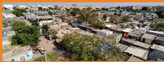
A large portion of the urban population in cities of the global South live under housing conditions that render them additionally vulnerable to the impacts of extreme heat (Image Credit: Goutham Raj Konda).
