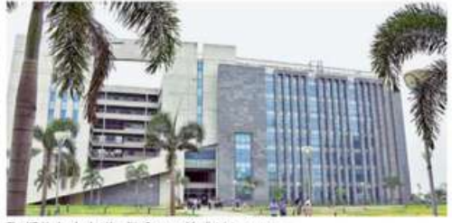
The IIT-Hyderabad at Kandi in Sangareddy district. *THE HINDU
