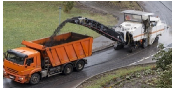
Figure-3: Milling of RAP material (Source: dykespaving.com)
