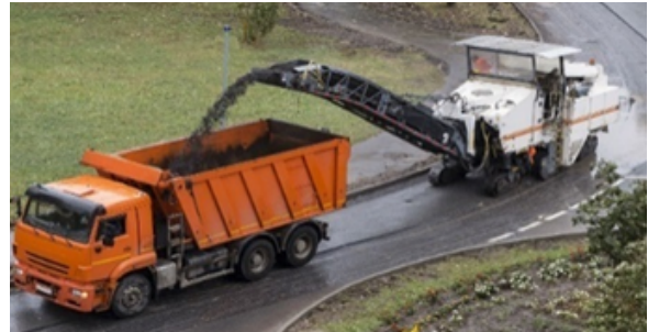
Figure-3: Milling of RAP material (Source: dykespaving.com)
